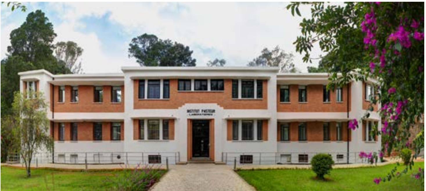
The Girard building of the IPM housing five research units
